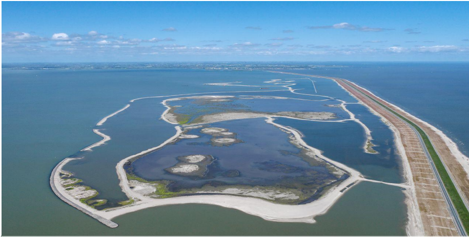
Cost-effective land water interfaces with 1) ability to adapt with changing forcing conditions and 2) opportunities for ecosystem enhancement.
